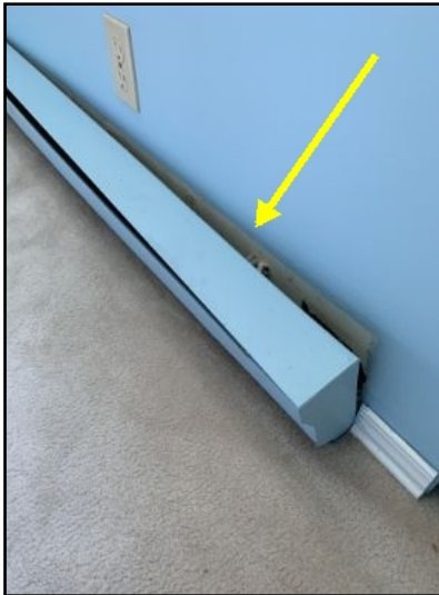
Secure baseboard heater to wall for safety
