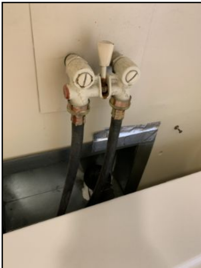
Replace rubber washer hoses with stainless braided lines to prevent hoses from cracking, bursting, leaking and/or possible future water damage
